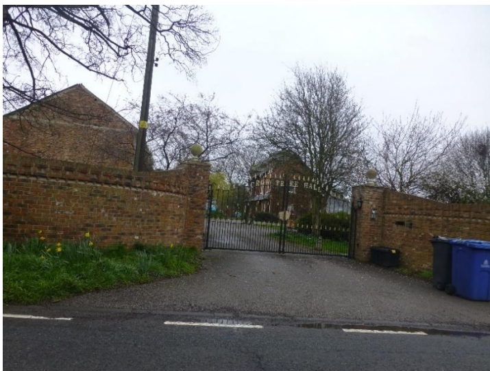
Plate 41: View of Crow Tree Hall looking east
